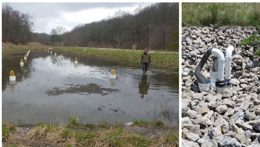
Fig. 4 (Left) Steel slag leach bed in East Branch of Raccoon Creek, Ohio. (Right) Periscope outflow structures to control air inflow to the underdrains of a steel slag leach bed. Photos by N. Kruse Daniels
