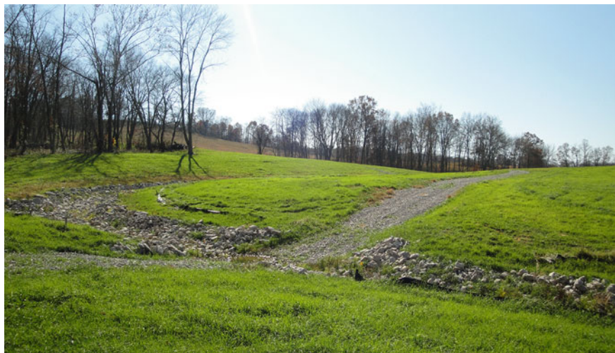
Fig. 5 Open limestone channel flowing from left to right forming the drainage structure from a reclamation project at Orland Gob Pile in Hocking County, Ohio. (Photo by N. Kruse Daniels)
