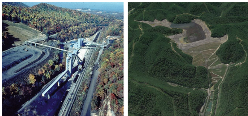
Fig. 7 A coal processing facility adjacent to a rail line (Photo by C. Zipper), and (right) a coal refuse disposal area occupying > 100 ha in southern West Virginia, with some refuse in the lower center of the photo having been covered with soil and revegetated. The dark-colored area in the photo's upper center is a coal slurry impoundment (Image from Google Earth)
