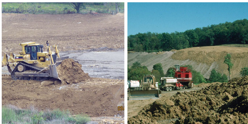
Fig. 3 A dozer spreading salvaged soil materials over mine spoil (left); salvaged soil storage piles (foreground, right) and a mine site backfill where salvaged soil has been partially applied (background, right) (Photos by Jeff Skousen)
