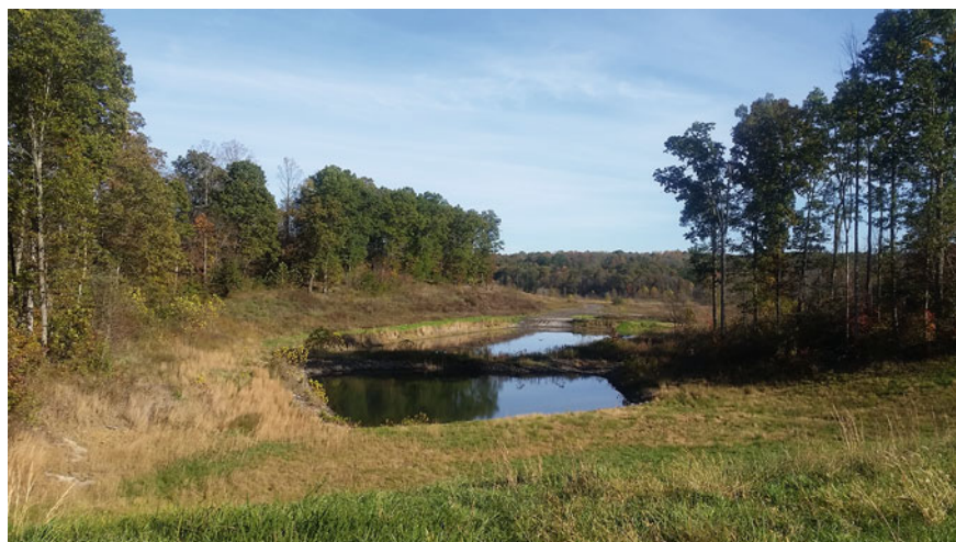
Fig. 6 Vertical flow reactor in the foreground serving as pretreatment for source water to a steel slag leach bed treatment system in the distance. Photo by N. Kruse Daniels
